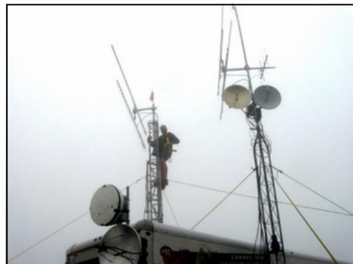
When the tower was re-erected, the rotor decided it was tired and we wound up with a 90 degree offset from the indicator. As there were some of the club’s older no-brake rotors, we needed Brian to **climb the tower** and reset the direction—the mission was accomplished quickly and we were back on all bands through 24GHz.
